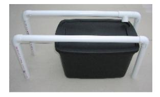
**9.** Next add the two 5" pieces to the bottoms of the legs. Glue one elbow on each end of each of the 5" cut pieces, making sure to seat them all the way in for each joint. Then glue to the bottom end of the two assembled frames. The two taller legs (18" and  $16-\frac{1}{2}$ ") go to one "U" and the two shorter legs (17 ½ and 16") go to the other "U". This is what it looks like all glued up:
