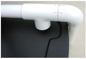
**8.** Next glue in the two shorter legs to the front rail, using the  $35-\frac{1}{4}$ ",  $16-\frac{1}{2}$ ", & 16" pieces. Do a dry run first, lay the assembly flat on the floor, and mark where the pipe goes into the elbows like below. Then glue them on. Push flat on the floor as you glue together so it is FLAT.
