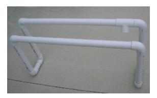
**10.** Now it's time to drill the drain holes in the back drainage rail (the one with the t-piece). Set the three Bato buckets onto the frame so they line up evenly between the elbow and the T-piece and mark on the PVC pipe where the drain holes come out:
